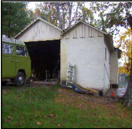
Before the project began, the “boat house” looked like this from the outside.
